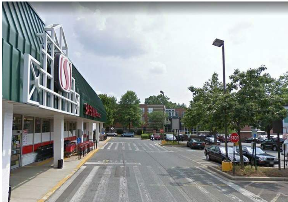
4. SAFEWAY BUILDING LOOKING SOUTH
